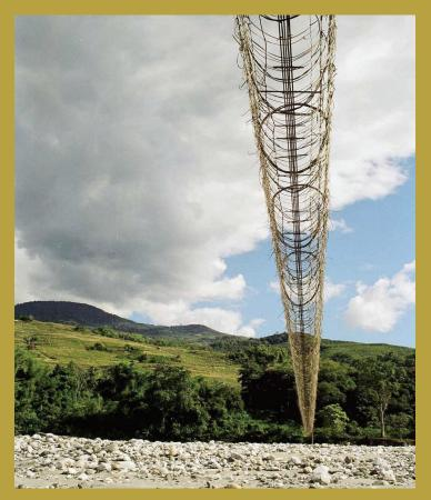
Built from traditional cane and bamboo, the bridge hangs across the Yamne River. Using canes and wires, it is held between suspension cables with a walkway made of halved bamboos for paneling used as protection. The use of these materials is also the mark of the local tribal culture. This 1000 ft. long suspension bridge is used by the tribal's to reach the other end of the bridge for their daily activities and livelihood.
